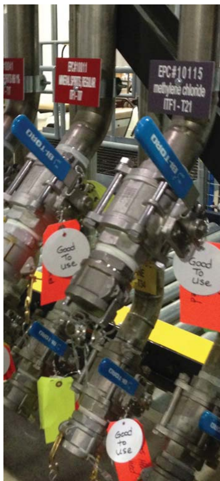
Outfitting a brand new chemical manufacturer's plant in 2012.
