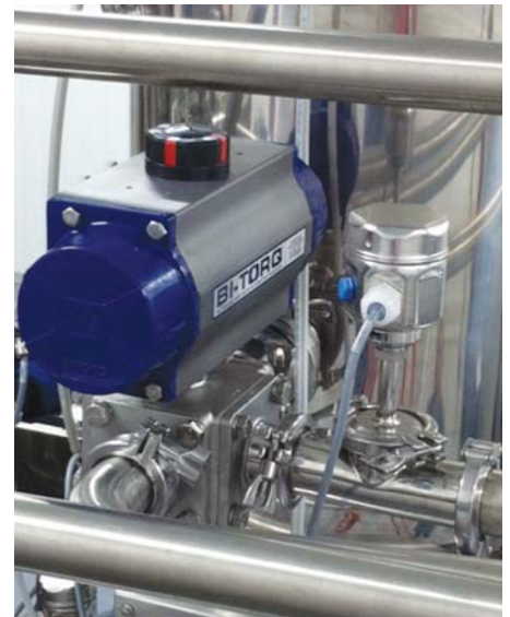
3-way sanitary ball valve on an apple sauce hopper.
